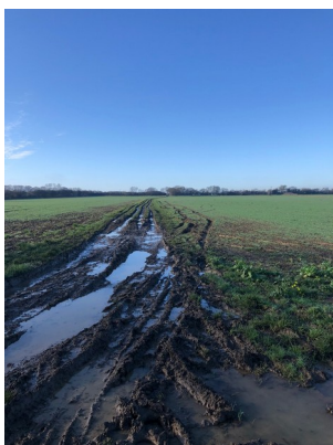
Recreational motor vehicle damage in 2020 to the Aston Cantlow unsealed unclassified road and adjacent arable land.
