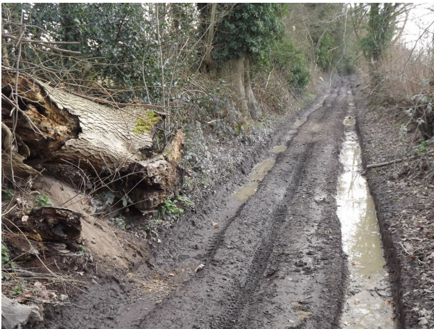
Photo © Colin Smith (cc-by-sa/2.0) 4x4 and motorbike ruts on Selborne BOAT in 2012, repaired by Hampshire County Council in 2017/18.
