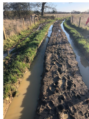
Recreational motor vehicle damage in 2020 to the Aston Cantlow unsealed unclassified road, now a bridleway.
