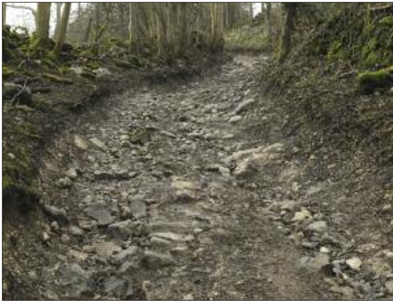
Brushfield as it rises from the Wye valley: enclosed, narrow with blind bends, nowhere to escape from oncoming vehicles and now badly damaged. Before use by 4x4s and motor bikes this was an easy route for horse riders and walkers.
