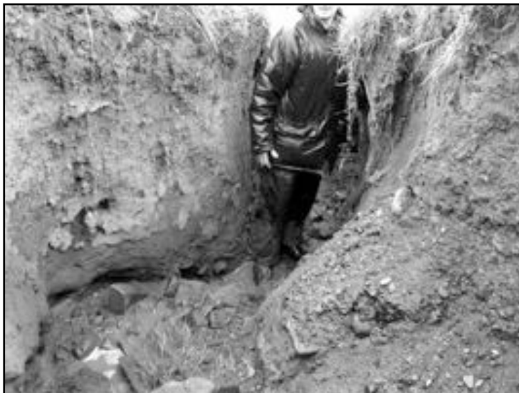
Chapel Gate (now being repaired by Derbyshire CC)
